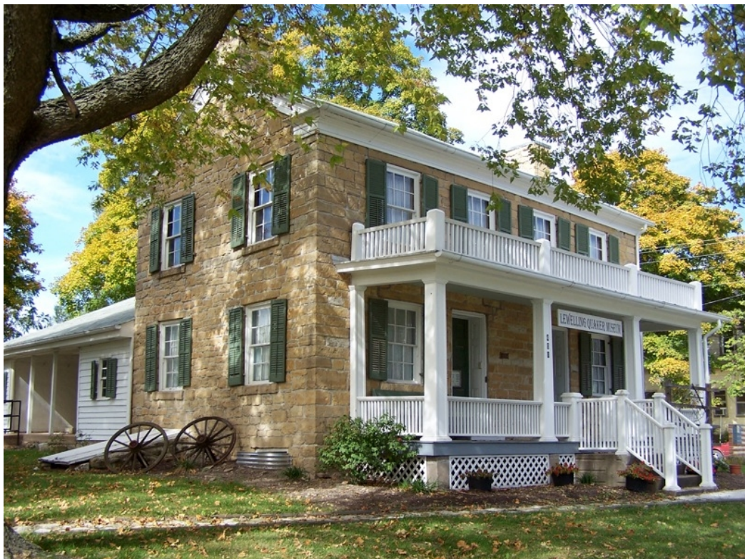
The Henderson Lewelling House, Salem, IA. (National Park Service)
